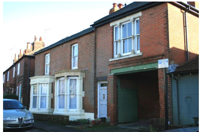
45 North Wallington –Formerly the Brewery Manager's House
