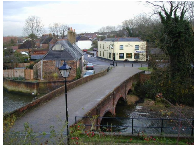
Wallington Bridge looking east into the conservation area
